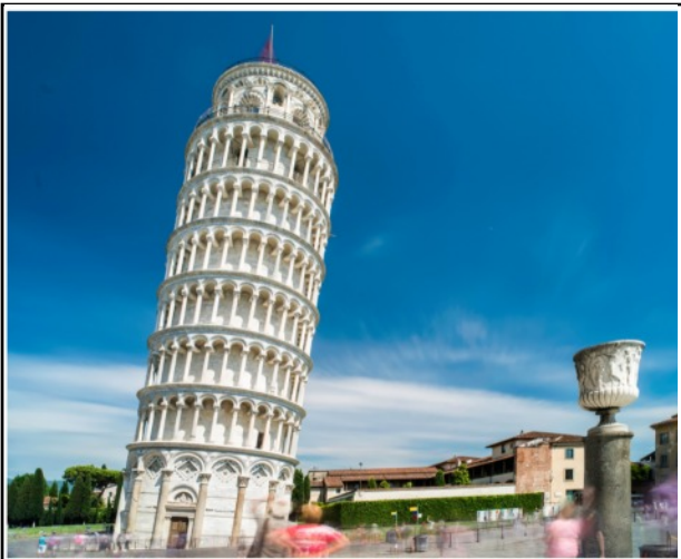
LEANING TOWER OF PISA
