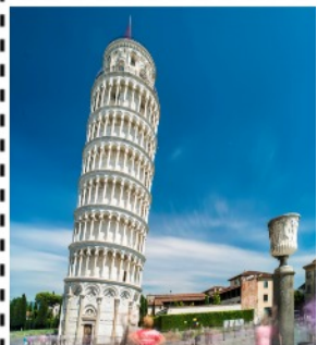
LEANING TOWER OF PISA
